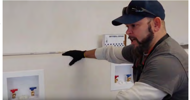
Hickman Mills electrician Felix Labrador surveys the work installing the Loads of Love laundry room.
