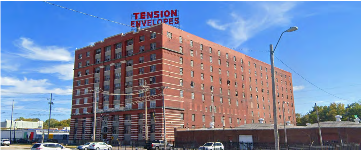
Tension Corporation's Kansas City office and manufacturing plant
